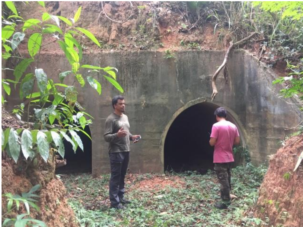
Inspecting an underpass that allows a giant armadillo to cross the highway
